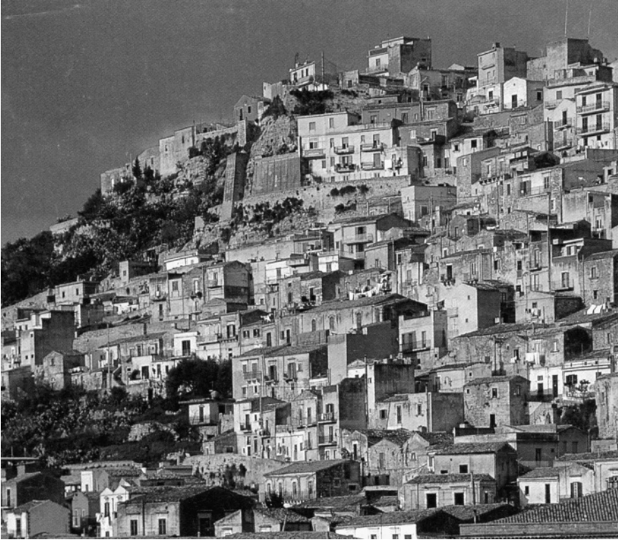
Figure 1.3 Illustration of hillside development that blends or fits into the terrain without excessive topographic disturbance.
