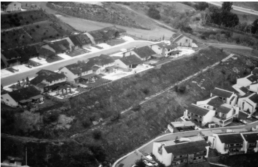
Figure 1.4 Transformation of natural hillside topography as a result of modern grading practices into two basic components, namely, flat pad areas and planar slopes.
