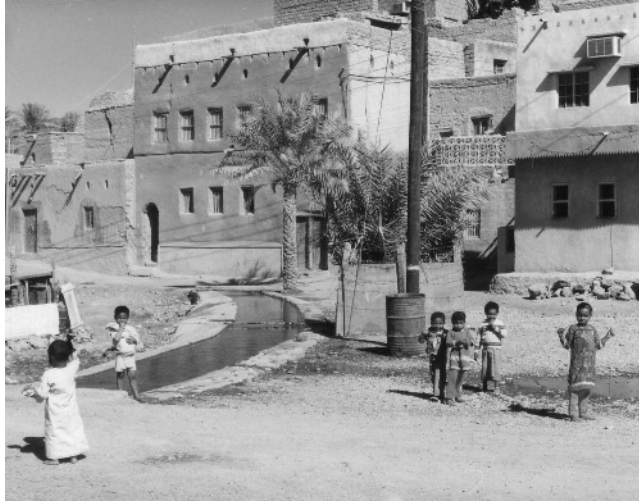
Figure 1.1 Open section of falaj (qanat) running through a village in northern Oman. Photo by Bruce Misstear
