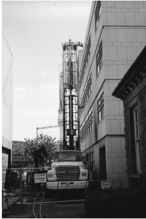
Figure 1.5 Drilling rig being set up for constructing a well in a gravel aquifer used as a source of geothermal energy, Dublin, Ireland. Photo by Bruce Misstear
