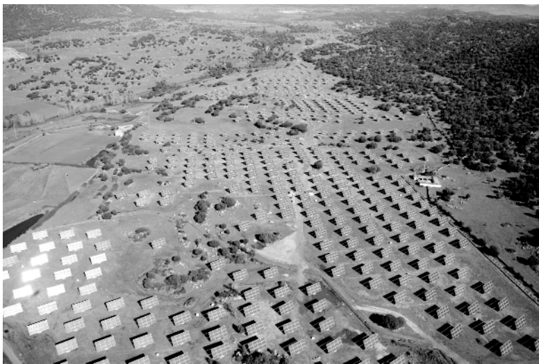
Figure 1.10 The Jerez de los Caballeros 10MW PV plant. Reproduced by permission of Guascor Solar SAW
