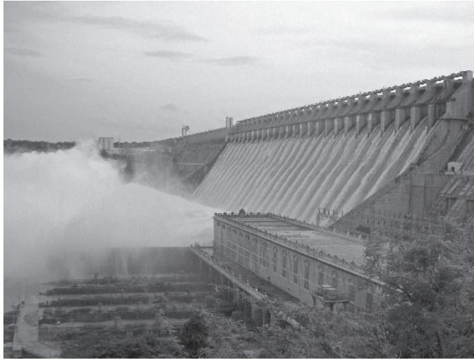
Figure 1.27 Hydroelectric power generators at Nagarjuna dam and hydro-electric plant, India. [Reproduced with permission from Wikipedia.]
