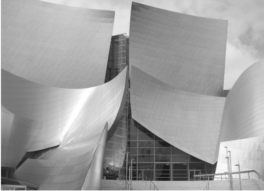
Figure 1-2 Example of cutting-edge projects, at the other end of the architectural spectrum from utilitarian works. Walt Disney Concert Hall. Alpen/Walker Images.
