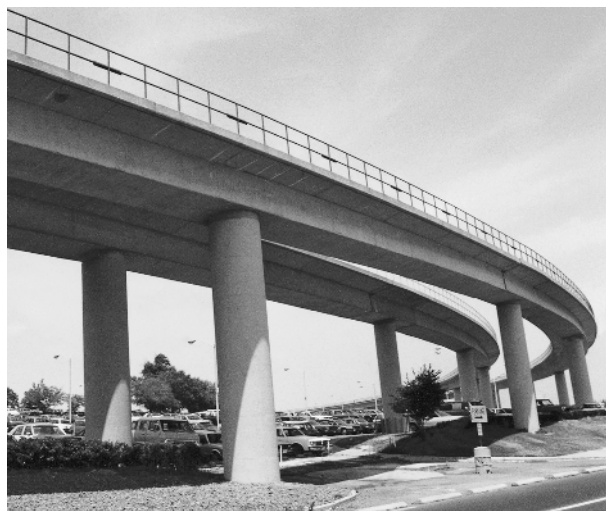
Concrete bridge for the city transit system, Washington, DC.
