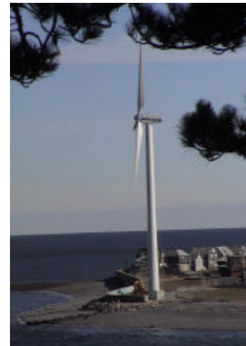
Hull's new 660kW wind turbine viewed from Peddocks
